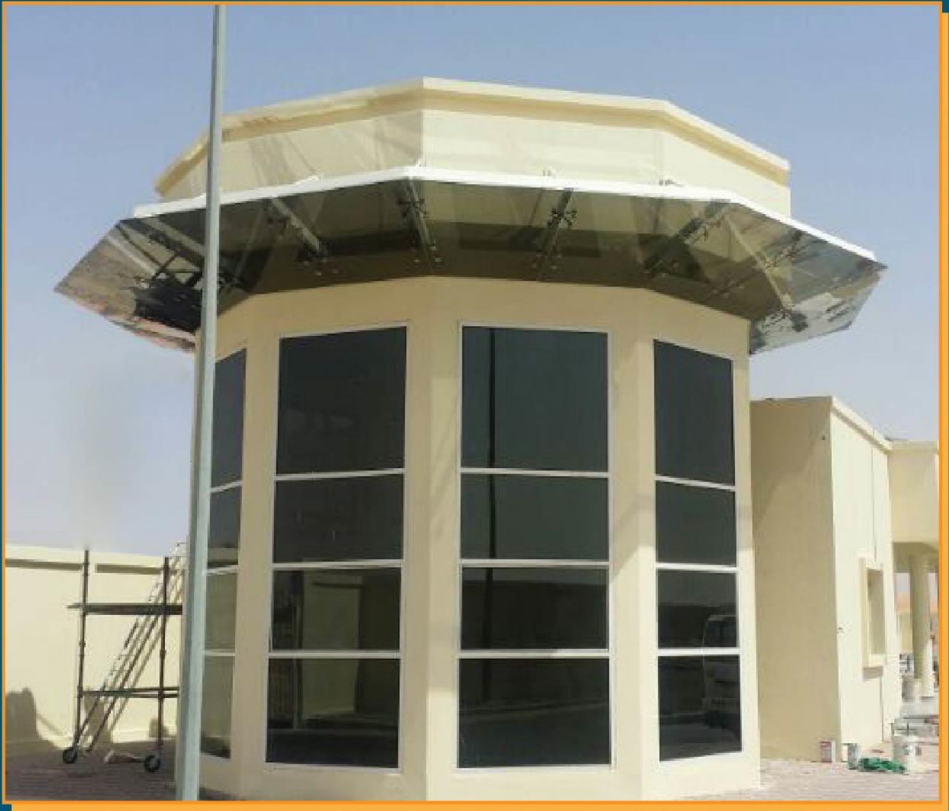
Sweihan Waste water treatment Plant capacity upgrade
