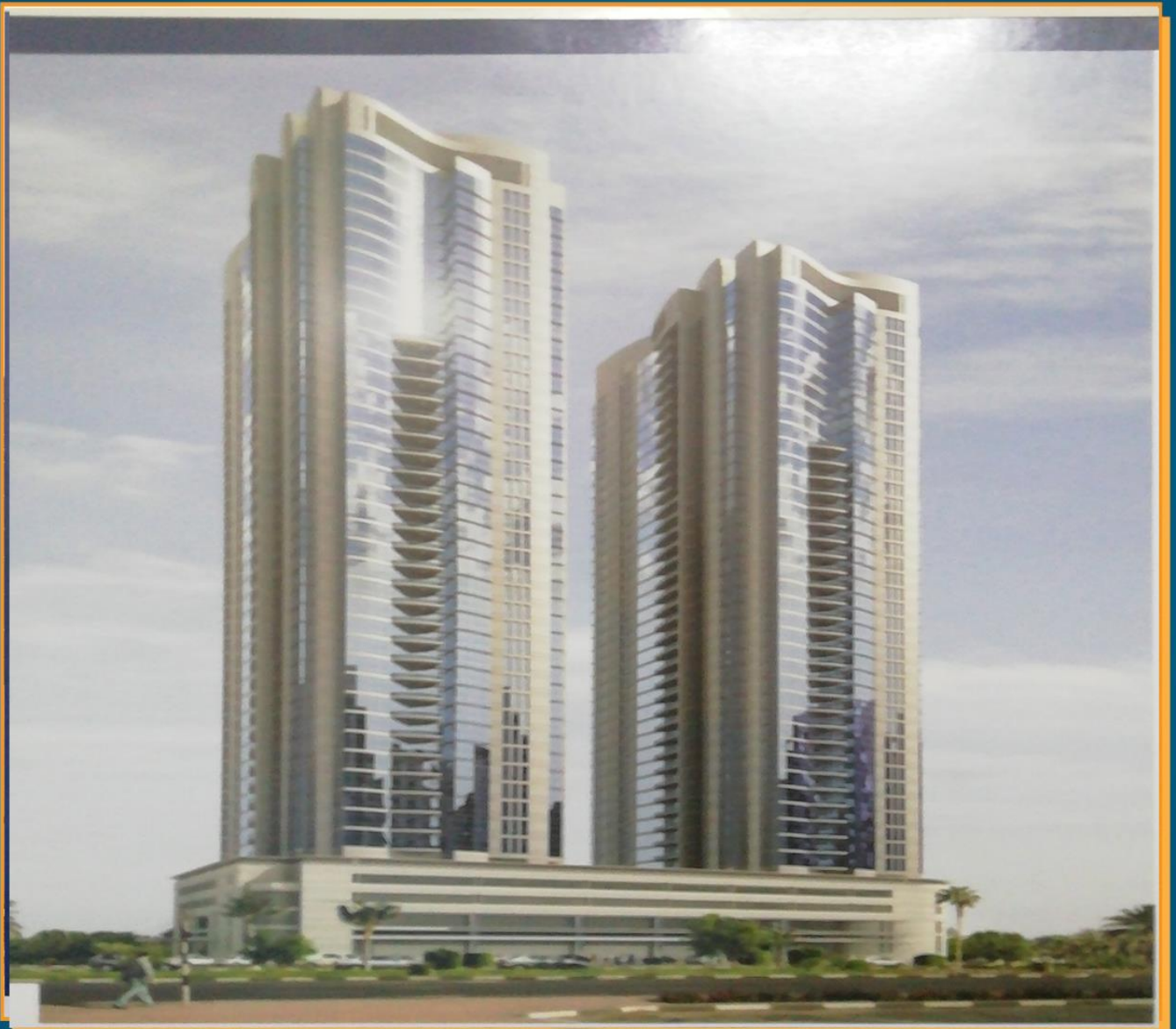
Sheikh Omer Bin Zayed Project, Abu Dhabi, UAE
