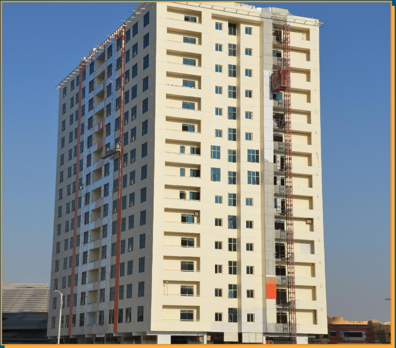
Building (B + C + 14 + Gyms)
